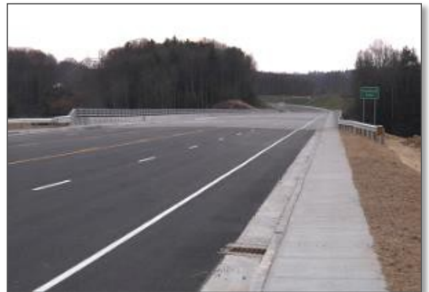
The design for the East Beckley Bypass included sidewalks and paved shoulders which now become part of the regional bicycle and pedestrian network.
